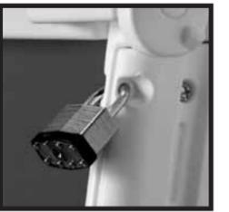
**OUTSIDE TREADS MUST BE IN THE UP POSITION AND LOCKED AT ALL TIMES WHEN POOL IS NOT IN USE.**
