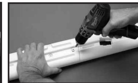
**#2:** Connect the Upper and Lower Outside Rails together using two #20 x 1/4" x 7/8" bolts and two 1/4-20 hex nuts. Repeat to assemble second Outside Rail.
