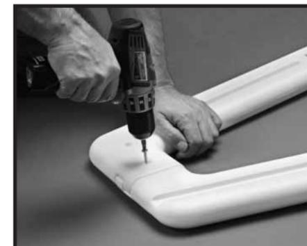
**#4:** Attach rails using two #10 x 1-1/4" self-tapping screws (one in the designated mark on the inside rail and one on the outside rail). Repeat for remaining return rail.
