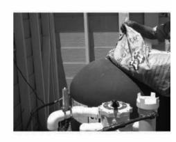
Step 6. Fill filter tank with the required amount of Zeobrite Filter Media. (Note: Zeobrite weighs 50% less than sand per cubic foot, therefore, it requires 50% less weight of Zeobrite versus sand.) See the Media Requirement Chart below.
