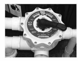
Step 9. After backwash, move multi-port valve to the rinse position and run until water clears in the site glass. Turn-off filter pump, move multi-port valve to the closed position and proceed to Step 10.
