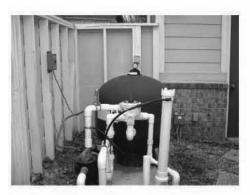
Step 1. Turn-off power to filter pump. Turn multi-port valve to the closed position. Clear work area and observe all safety precautions. For new filter installations, skip to Step 5.
