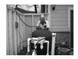
Step 5. After removing sand, rinse and clean filter tank. Inspect laterals and piping for defects, repair if needed. Inspect multi-port valve for proper operation. Replace drain plugs and fill bottom 1/3 of filter tank with water.
