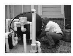
Step 3. If filter is equipped with a drain plug, remove drain plug and drain water from filter tank.
